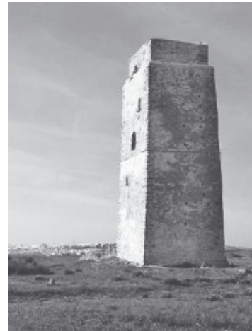
A neglected ruin Exterior view
